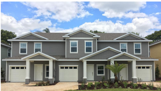
Atrium Management built about 40 multifamily homes in downtown Orlando's Milk District.
